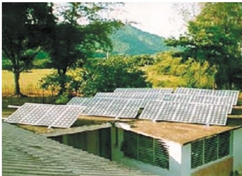
Solar PV Installation in rural Cuba
