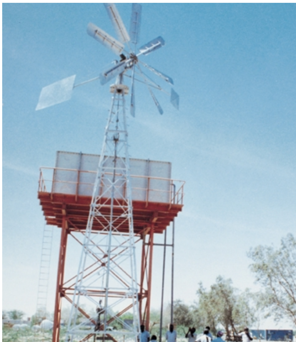
Locally-manufactured wind pump installed at kilo 8 site
